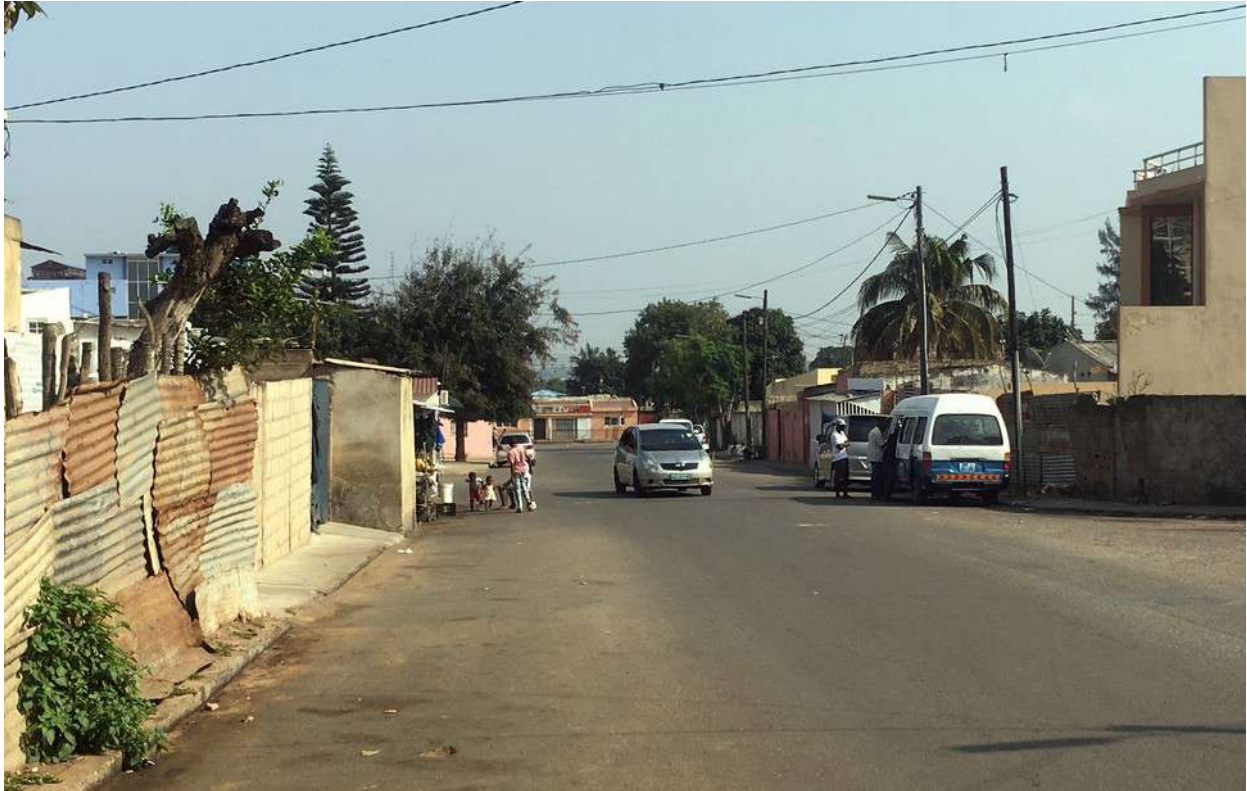
Figure 64: Newly paved street in Maxaquene B neighborhood (Maputo City). Source: Romero
