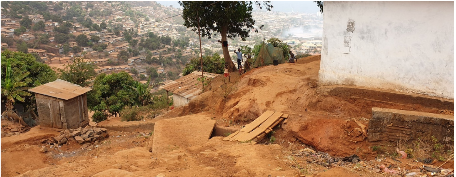
Figure 8 Constructed Bridge in Moyiba. Source: https://www.walkingcitieslab.com
